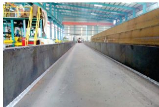
Welding by pull through machine
