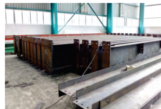
MIG Welding for connection plates & stiffeners
